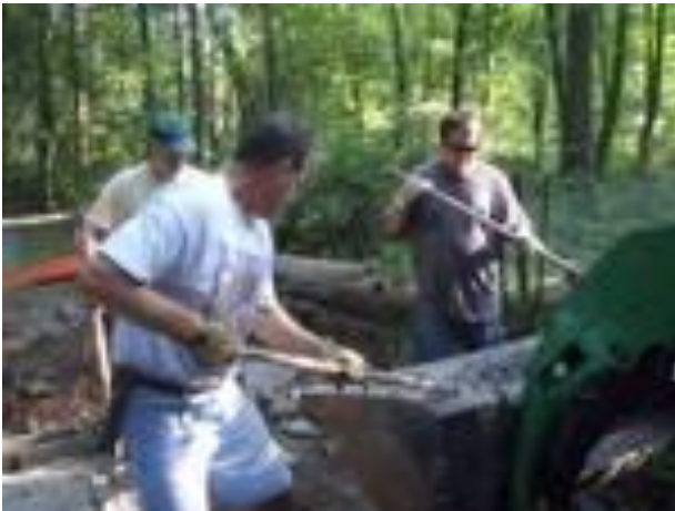
Figure 1-Gary, Hamp & Scott mixing concrete in the bobcat bucket.
